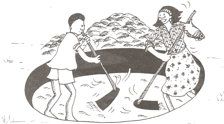
Figure 4.2 Digging the foundation
