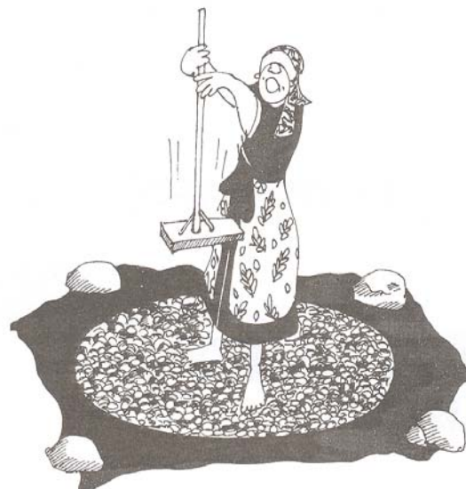
Figure 4.4 Levelling the foundation
